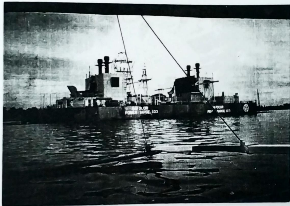
PLATE 6 THE NAPOCOR POWER BARGE A POSSIBLE POLLUTANT
